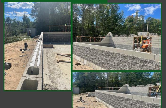
Description: The village of Roscommon needed a new wellhouse. Omni Block was chosen because of its lower cost when compared to a standard CMU wall.
