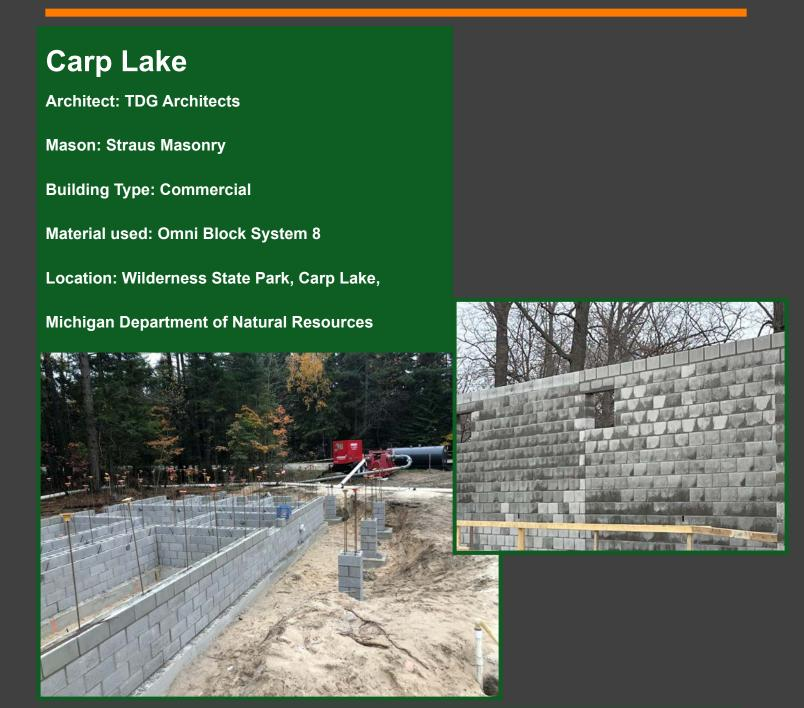
Description: Omni Block was used on this project because of its ability to hold in heat. This is due to the design of the cross webs that don't allow for Thermal bridging. The added benefit is the cost reduction as there is no need for materials such as furrings and sheetrock to meet the energy code.
