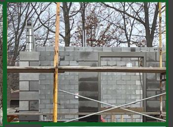
Description: Kent County utilized Omni Block for this pump house which is located in a neighborhood. They used Omni Block for the building and then added siding to ensure the pump house blends in with the neighborhood.
