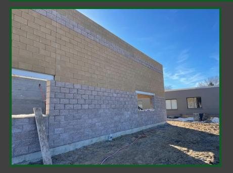
Description: Hope Protestant Reformed Christian School utilized Omni Block for an addition onto the pre-existing school to be used as a music room. Omni Block was chosen because of its ability to meet the energy code in a single-wythe wall and its ability to stand the tests of time.
