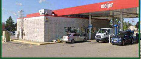
Description: Meijer has used Omni Block on a few different gas stations. The higher R-value and fire rating is perfect for gas stations as it is reliable and lowers the cost as compared to a standard CMU wall. The fire rating for Omni Block System 8 is 2.3hr and the fire rating for Omni Block System 12 is 4hr.
