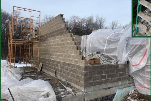
Description: Omni Block was utilized for this job because of the ability to use a single-wythe wall and still meet the energy code while being a masonry building that has a far longer life than timber.
