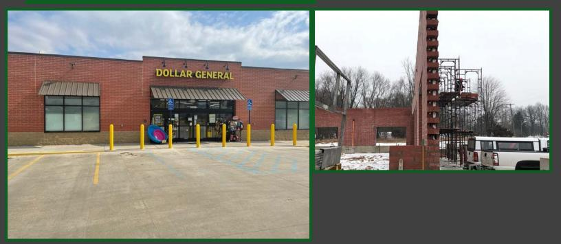
Description: The city ordinance for Alto, MI required the building to be built out of CMU and brick. Omni Block was chosen because of the energy savings and cost savings that are associated with using fewer materials.
