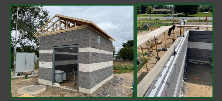
Description: The city of Holland needed a pump house built that will stand the test of time while also reducing the amount of energy needed to maintain. Omni Block was a great pick because of its high R-value in a single-wythe wall less material was needed to build and meet the energy code.
