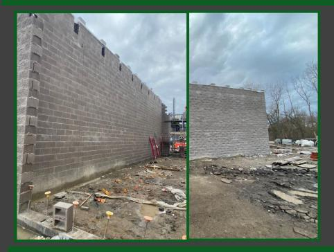
Description: Northville decided to utilize Omni Block because of its high R-Value. The Transportation building is open year-round which means they use a lot of energy annually for the building. Utilizing Omni Block reduces the amount of energy that is used since the building can maintain temperature with no Thermal Bridging.
