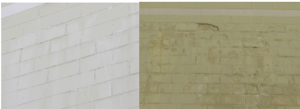
Figure 8: Section of wall worsening over time from 2011 (Left) to 2017 (Right)
