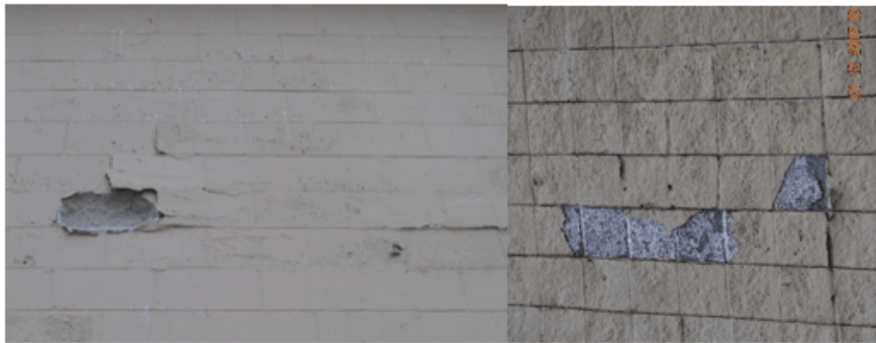
Figure 7: Excessive Peeling, Efflorescence, Cracking, and Spalling originating near roofline
