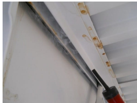
Figure 2: Smoke escaping at Roof/Wall Junction
